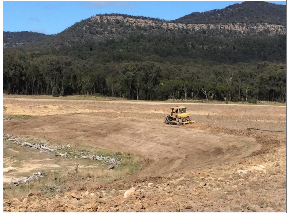
NWCD Rehabilitation Rework – Deep Ripping – 24/09/2015
