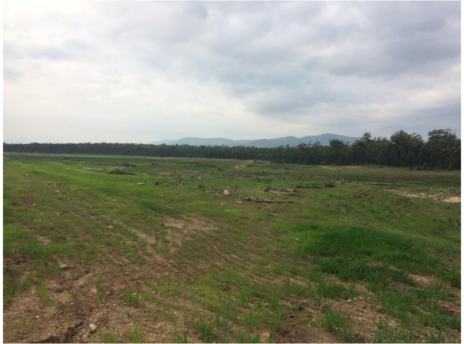
NWCD Rehabilitation Rework – Rehab Progression – 26/01/2016
