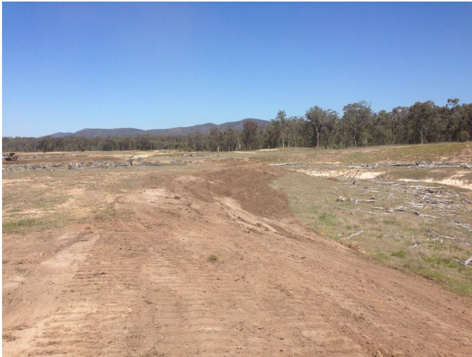
NWCD Rehabilitation Rework – Galenia Scalping – 11/09/2015
