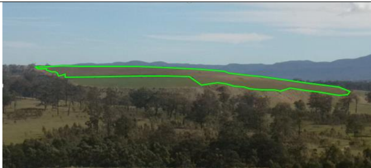
West Pit Out of Pit dump facing south-west across New England Highway – August 2016
