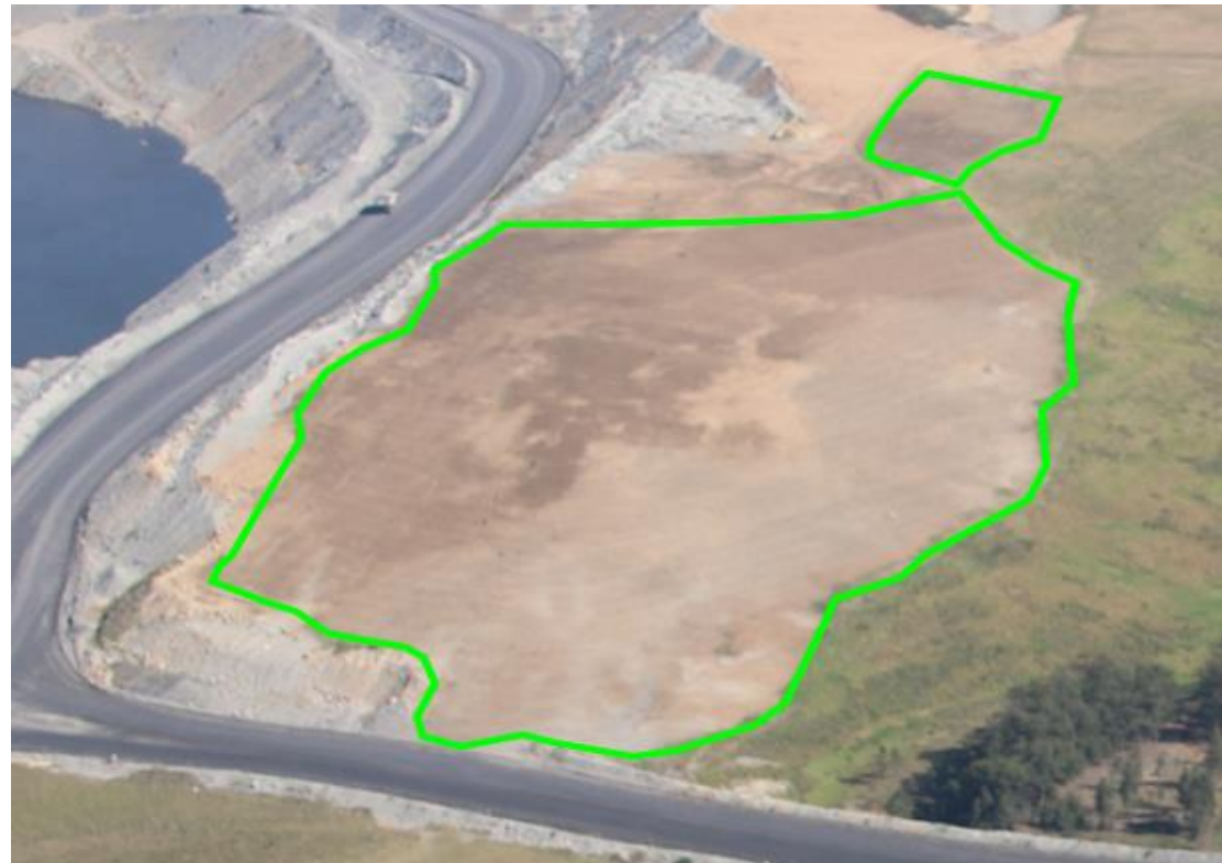
RCS - Arties Pit dump facing north-west – photo taken while spreading topsoil over subsoil
