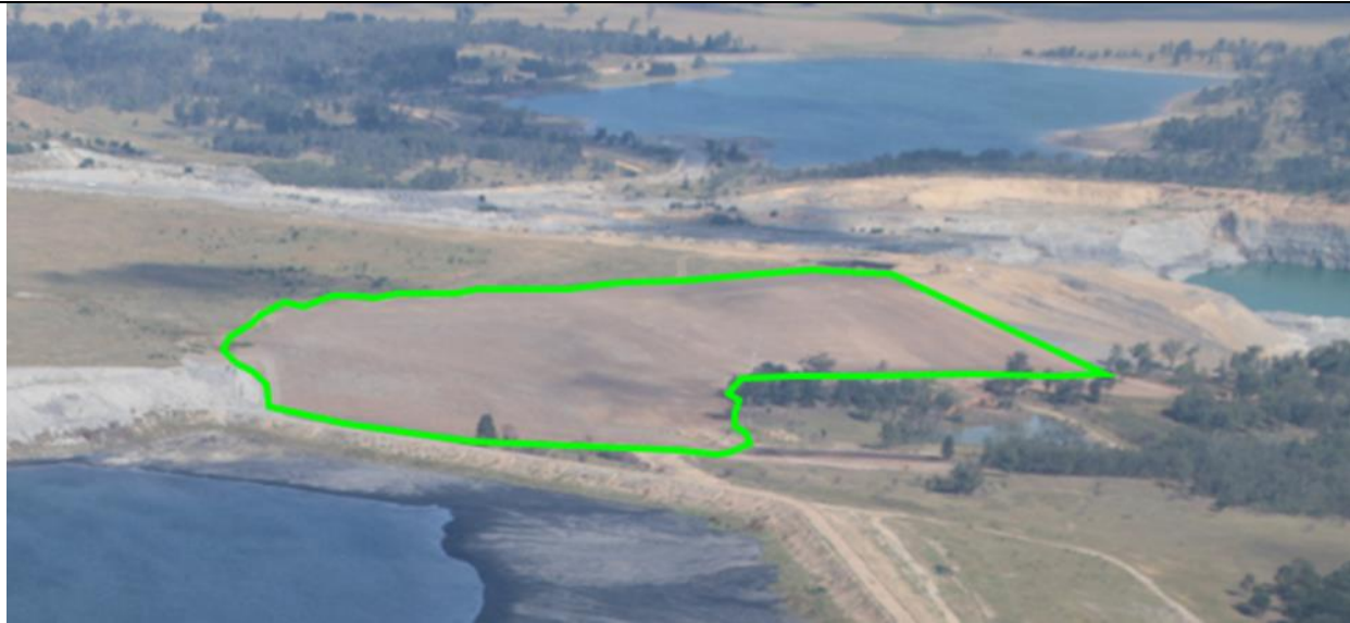
RCN - Falbrook Pit – Stoney Creek Road batter rehabilitation facing west
