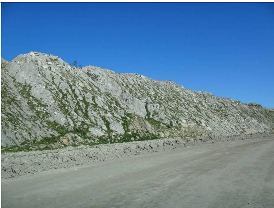
Aerial seeding on South Pit dump batters (3 months)
